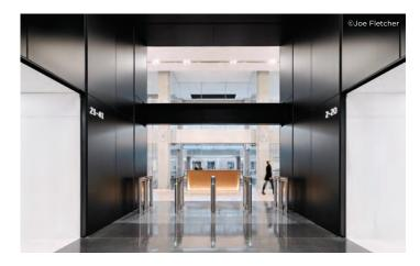
Laminated black glass panels, etched for light diffusion, are mounted with seismically-rated CaptiveHook®, providing contrast to the ethereal delicacy of the textured white walls.
