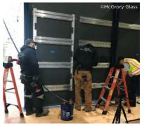
The plug-and-play system delivers fully manufactured panels that arrive on site ready for clean installation. Any piece of glass can be safely removed at any time, for any reason (including post-install maintenance), and easily replaced.
