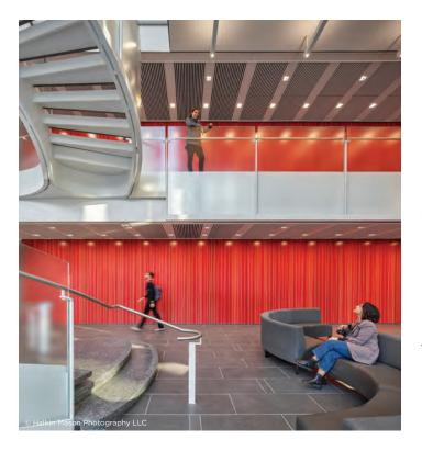
The McGrory team delivered 152 unique glass panels, each measuring 3' by 9'5", which encapsulated multiple unique elements and provided curved, acid-etched railing panels and 46 marker boards in various sizes.
